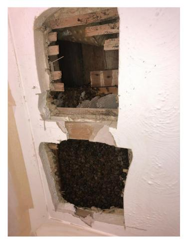
The four different layers of ceiling illustrate the work that has taken place on the ceiling during the lifetime of this property. The top layer was modern plasterboard, then foam, hard plaster and finally the original lathe & plaster layer. All of which the jigsaw had to cut through.
