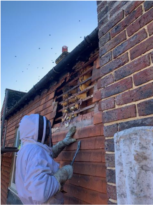
Vic about to remove the next row of tiles.
